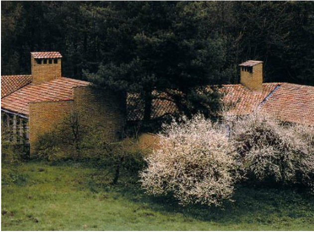
33 Kingo Houses 1956 Architect Jorn Utzon
